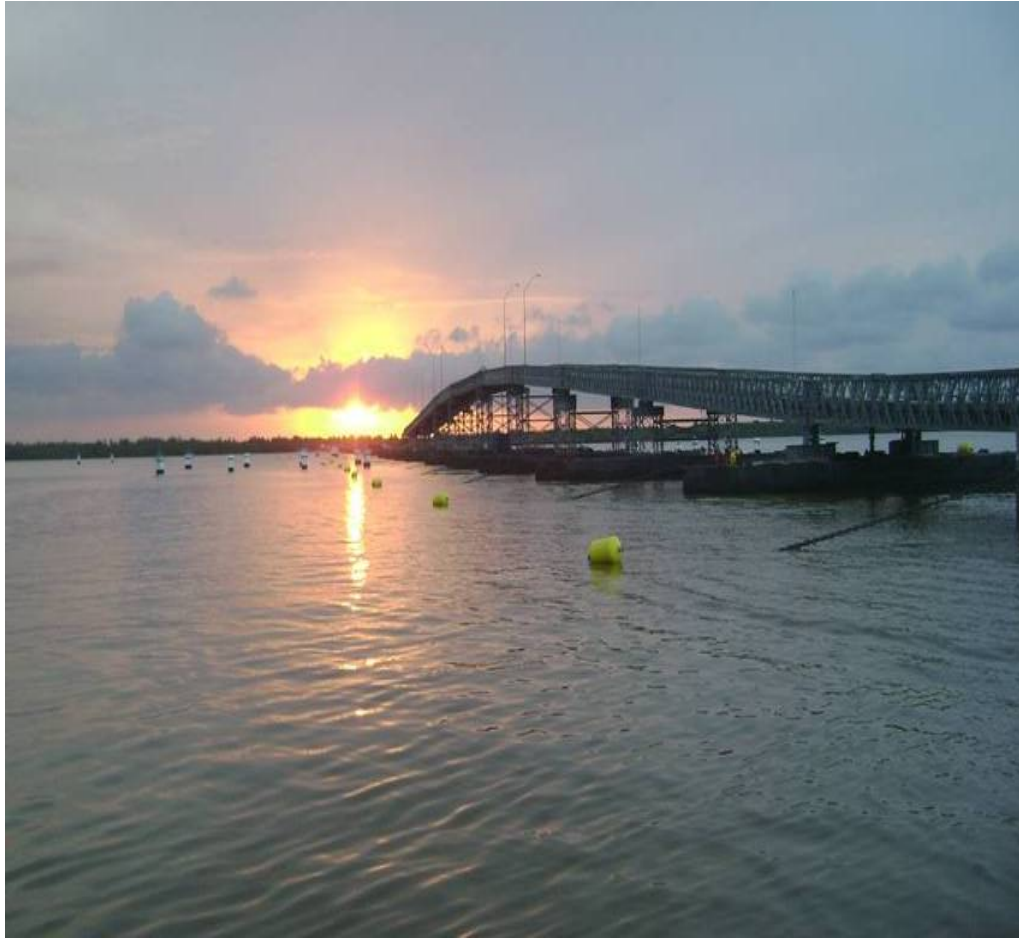
Figure 12 The Berbice River Bridge, in Guyana, SA
