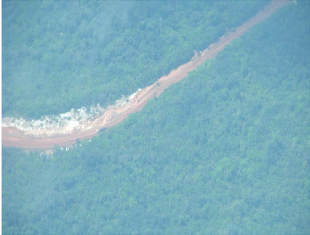
Figure 8 Road Transport on the Linden Lethem Road in Guyana
