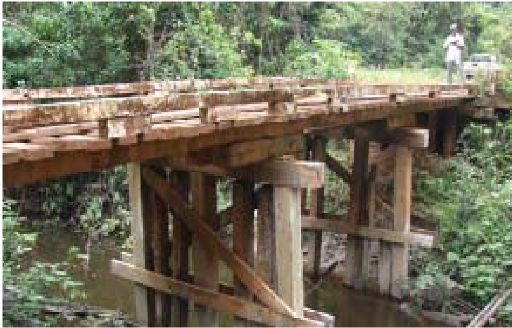
Figure 14 Bridge at Annai along the Linden / Lethem Road in Guyana
