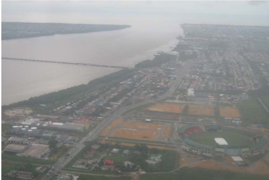
Figure 13 Demerara Harbour Bridge in Guyana, S.A
